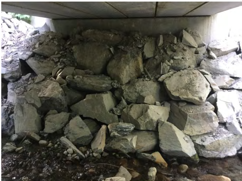
Left Bank Abutment when facing downstream
