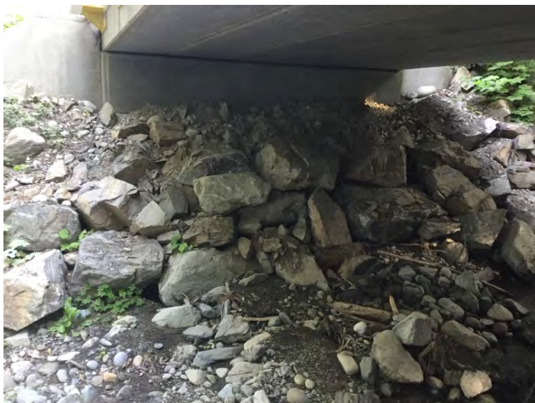
Right Bank Abutment when facing downstream
